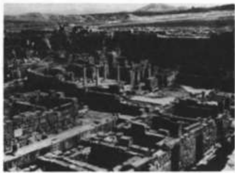
PLATE 19.13 Timgad (Algeria): Byzantine fortress, 6th century: south rampart, officers' living quarters and chapel
