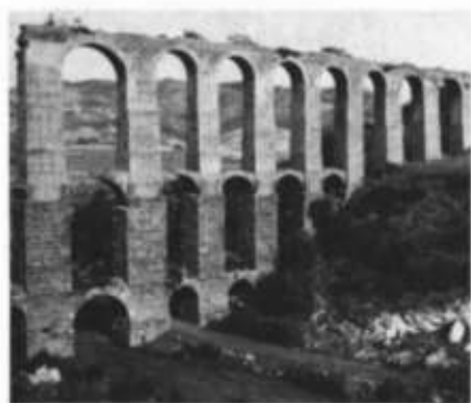
PLATE 19.3 Aqueduct from Zaghouan, which supplied Carthage
